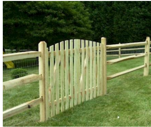
Wooden post with gate
